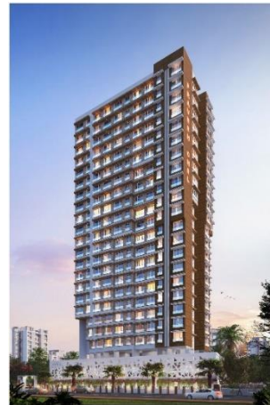
Pravesh CHSL – Borivali (E); 149,830 sq. ft.; Time Completion – 39 Months
